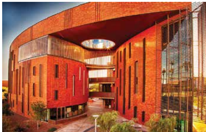
McCord Hall at Arizona State University W.P. Carey School of Business was a nominee in the 2016 ACI Excellence in Concrete Construction Awards
